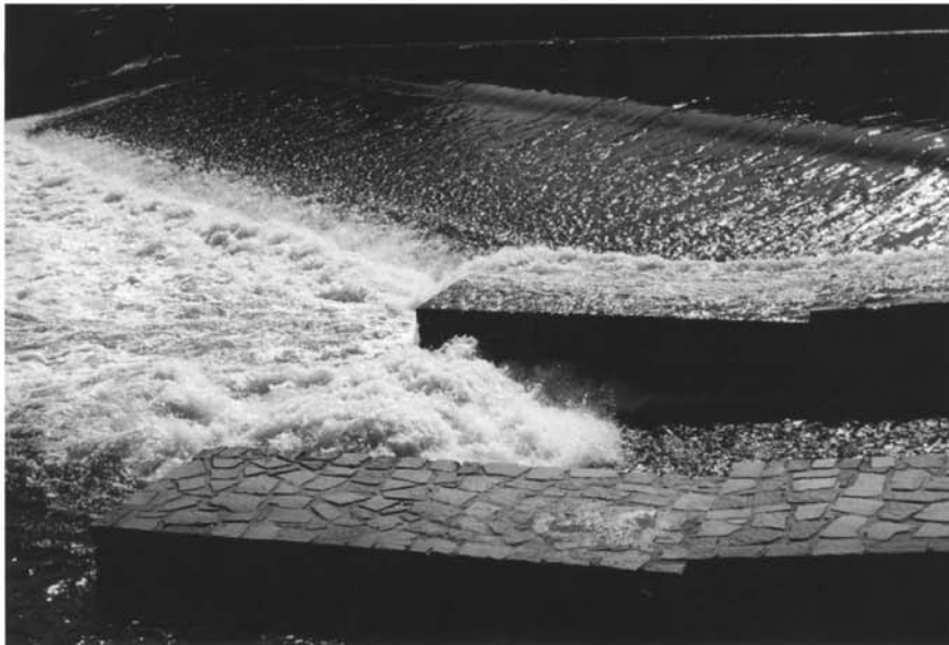
Figure 6.5. Hydraulic jumps. (a) A free-surface undular jump over a shallow ridge in a river flowing from right to left. The undulations – the waves – are stationary and those on the far side of the river are breaking along part of their crests, losing energy to turbulence. (b) Hydraulic jumps in the lee of a weir. The flow is from right to left, and the water in the sloping channel on the lower right of the photograph is shallow, about 0.2 m deep upstream of the breaking jump that creates foam and throws up spray. (c) An apparently stationary internal hydraulic jump in the stratified flow of air (from right to left) over the Sierra Nevada mountain range, visible at the left, in the USA. The jump is made visible by dust raised by the wind flow over the ground and by the formation of clouds. (Photograph by Robert Symons. Reproduced with kind permission of Professor R. S. Scorer.)
